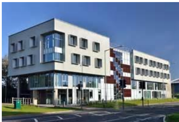
Figure 7: Picture of the ALLIA Future Business Centre
